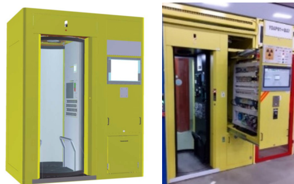
Figure 2: SPS PPS Personnel Access Device.
