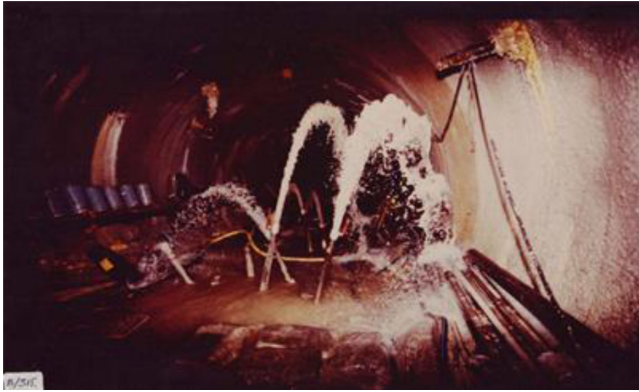
FIG. 23. Photo of water input to LEP tunnel.
