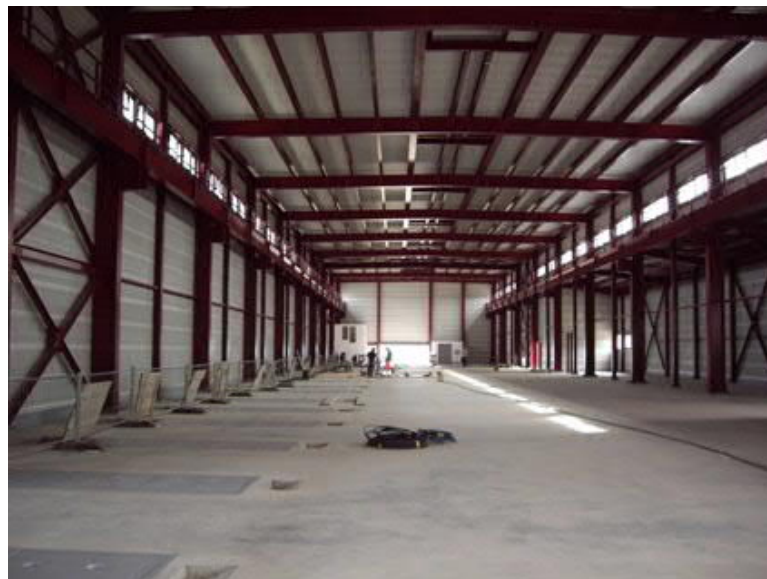
Fig. 4.7: Klystrons building steel structure.
