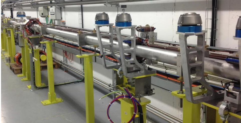
Fig. 2.25: L4T supports and survey target arms.
