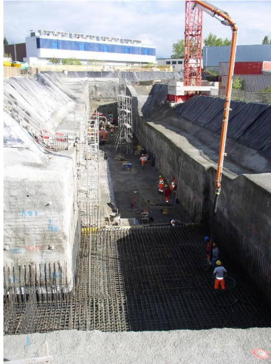
Fig. 4.4: Linac4 tunnel excavation works.
