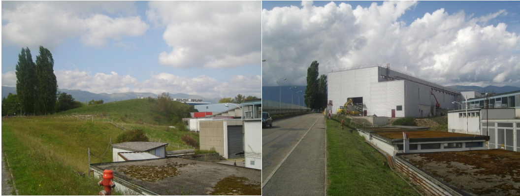
Fig. 1.2: Mount-Citron in 2008 (left) and the same position in 2010 (right), after construction of the Linac4 building.
