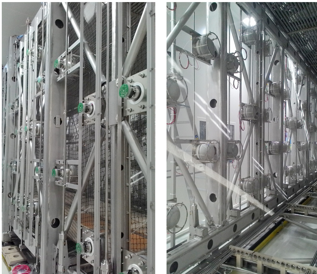
Figure 11. Picture of the PMT supporting system.
