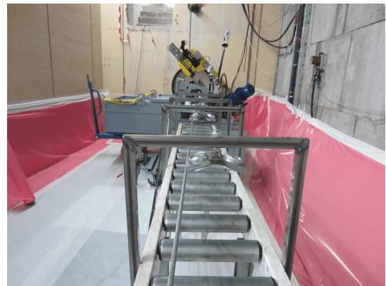
FIG. 17. Tooling for the extraction of the original dump core and beam pipe out of the dump cavity. In the foreground, the support structure with rollers and the winch cable. In the background, the remotely operated saw and the lead-shielded container.
