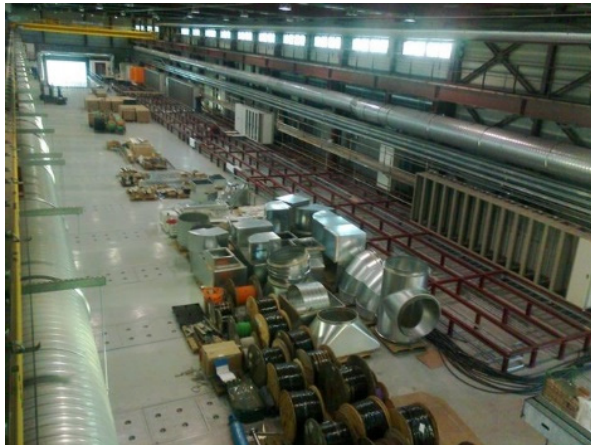
Figure 3: Linac4 hall during the general services installation.
