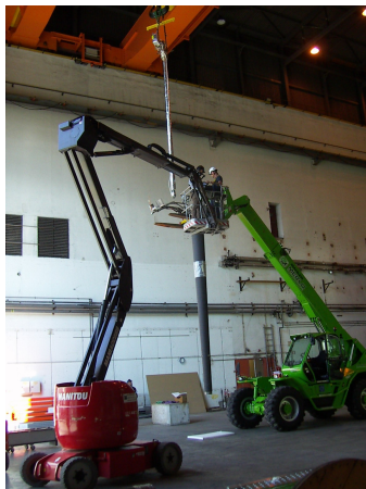
Figure 5. The installation of the beampipe into LUCID and the support cone.
