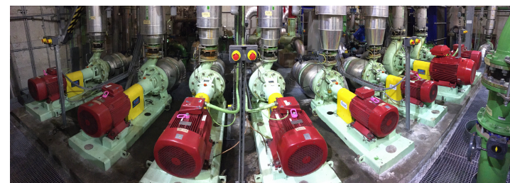
Compressors of the ID Evaporative Cooling System
