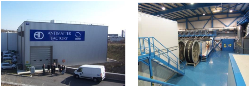
Fig. 6. Outside and inside the new building 393 — the Antimatter Factory — housing the kickers and storage place for the experiments.
