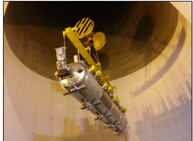
Figure 1: The spare RF cryomodule (four cavities) being lowered down into the UX45 cavern (Feb. 2014).
