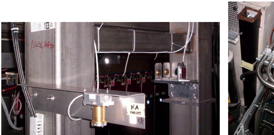
Figure 9: A CCD camera of a long vertical RASNIK line mounted on the bridge (left). A lens and a mask fixed together to the bunker's wall (right).
