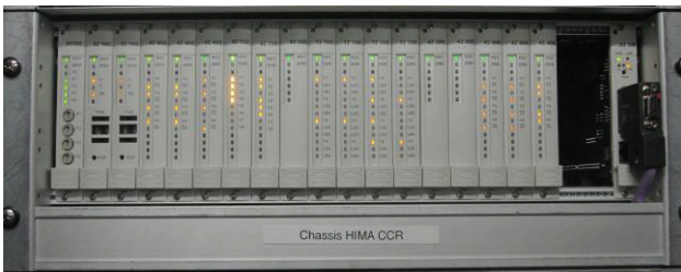
Figure 4: Planar4 wired logic in a 19-inch sub-rack. From the left: fuse module, two timing modules, logic modules, and far right a Profibus supervision module.
