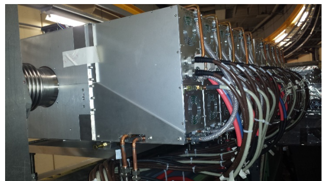
Figure 1: Prototype Finemet cavity modules installed in Ring 4 of the PSB.
