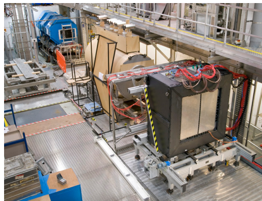
Figure 3. The EMR detector installed in the MICE Hall at the end of the preliminary ('Step I') beam line. The photograph also shows Q7–9 and TOF1 at the top half of the frame. A model of one spectrometer solenoid was positioned in the hall to allow installation procedures to be developed.
