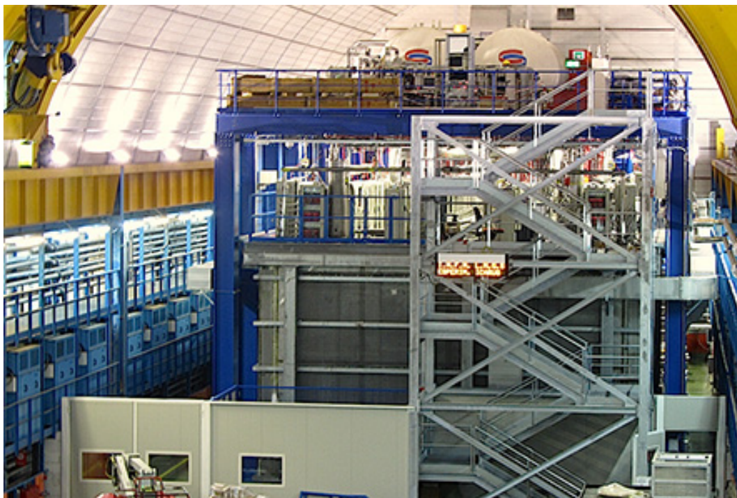
Figure 1. The ICARUS T600 plant in the Northern side of the Hall B at LNGS. Ladders to access the intermediate and the top levels are visible in the front together with the 3 m high wall that separates the T600 area from the rest of Hall B. Cabinets with the readout electronics are installed at the intermediate level. At the top level, the two 30 m 3 cryogenic storage tanks and the additional electronic equipment (HV supply, PMT electronics, trigger system, etc.) are also visible. The cryogenic equipment (nitrogen and argon pumps, cryocoolers, etc.) is located on the rear side of the T600, at the Northern end of the Hall B.
