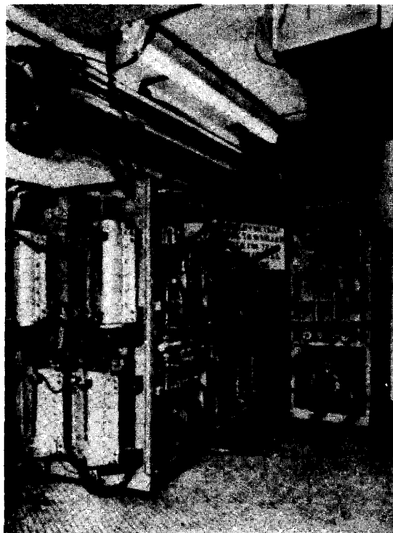
Fig. 14. Bending magnet pulse generator. Front left: Ignitron rack. Behind that: Capacitor bank. Right: Ignition and bending magnet temperature control.
