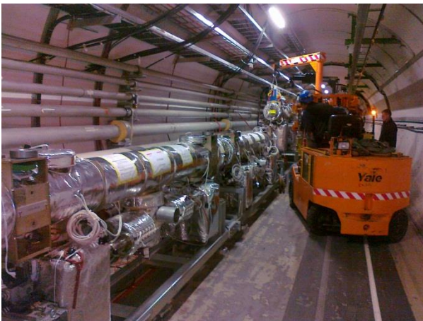
Figure 2: Installation of the last TCDQ tank on the movable girder.
