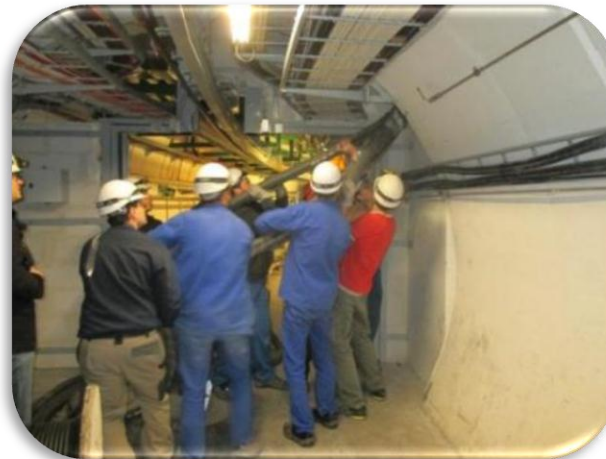
Warm Cable installation @ P5
