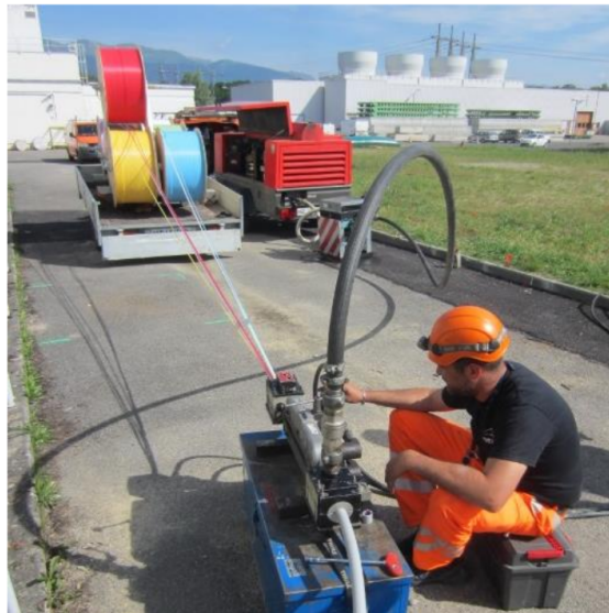
Figure 10. Optical cabling installation.
