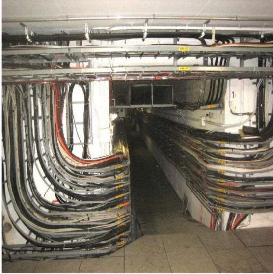
Figure 1. Cabling installation in the PS tunnel.
