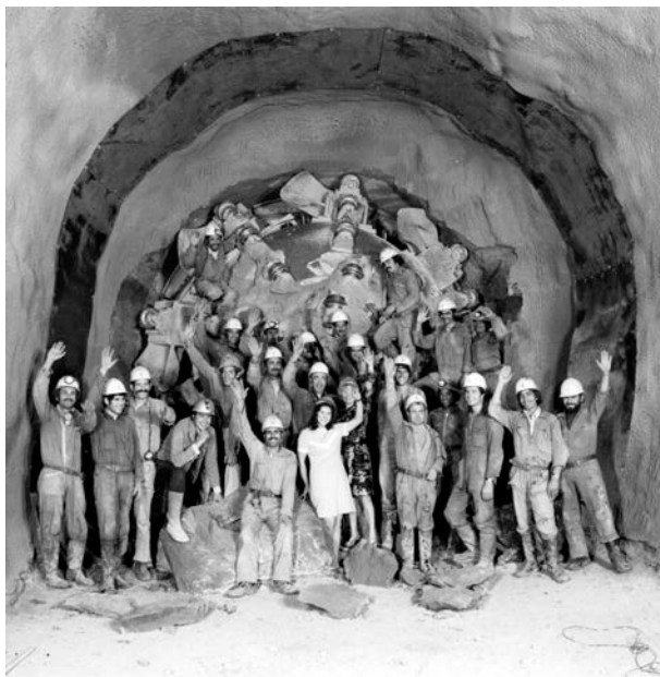
Fig. 15. Completion of the SPS tunnel excavation in 1974.
