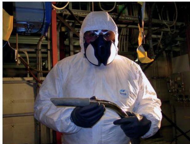
Fig. 9: Staff wearing protective clothing during work with SF 6 waveguides
