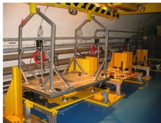
Figure 4: Photo of a support interface plate being positioned in the experimental area.
