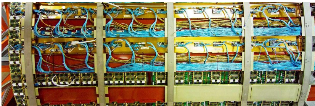
Figure 20. Partially assembled End Cap showing two full cable trays at the top and one empty cable tray at the bottom. Each tray carries cables for 1/32nd of the detector and acts as part of the outer Faraday cage of the detector. The blue cables are the 36 AWG data and control shielded twisted pairs, the heavier orange-brown cables are low-voltage supply cables. The light colored HV cables are just barely visible in the upper tray on the left. In this view the Triplet Boards serving the A type Wheel nearest the interaction point are on the left and the PPF1 connectors are just out of the picture on the right.
