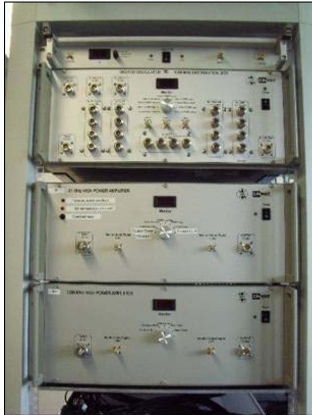
Figure 9.9 Frequency generation and distribution boxes
