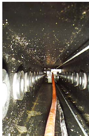
Fig. 22. A view of the inside of the Girder during the cutting and polishing process.
