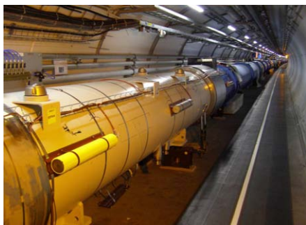
Figure 3: The location of the BLMs outside of the cryostat at the plane of the vacuum chambers. At the LHC arc two detectors are on the quadrupole magnets (white) and one on the adjacent bending magnet (blue).
