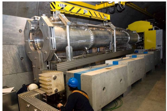
Fig. 6. The CNGS horn during installation.
